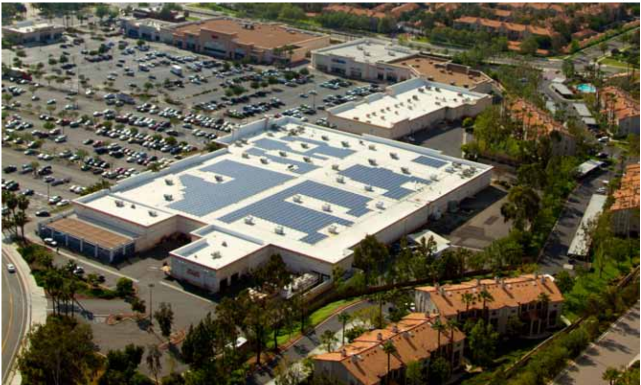
A Walmart location uses solar panels to generate power in Corona, CA.
